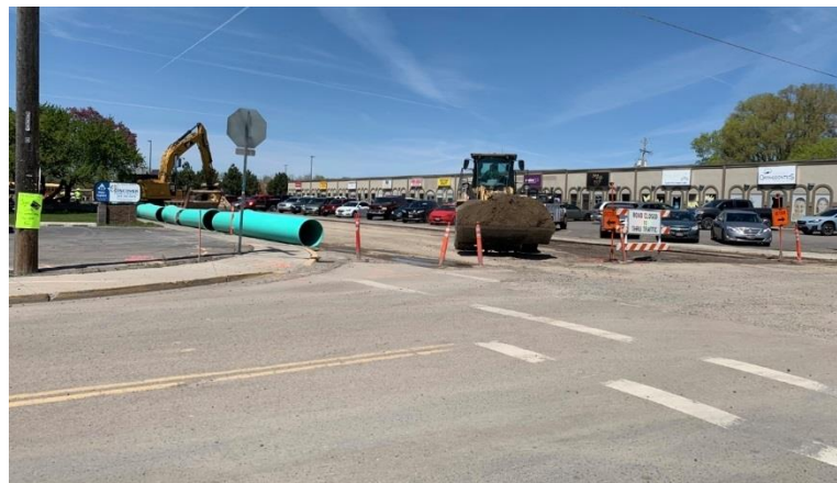
Street construction project
